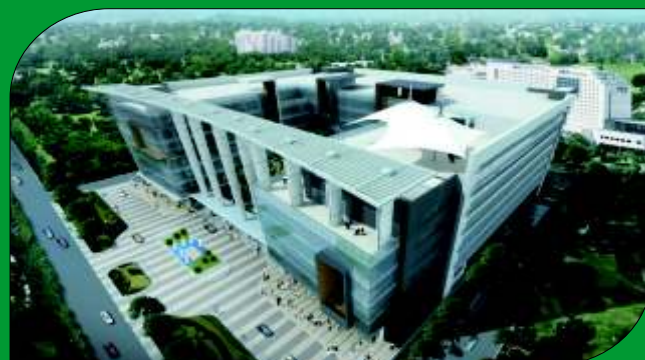
BPTP - I Park - Gurgaon
